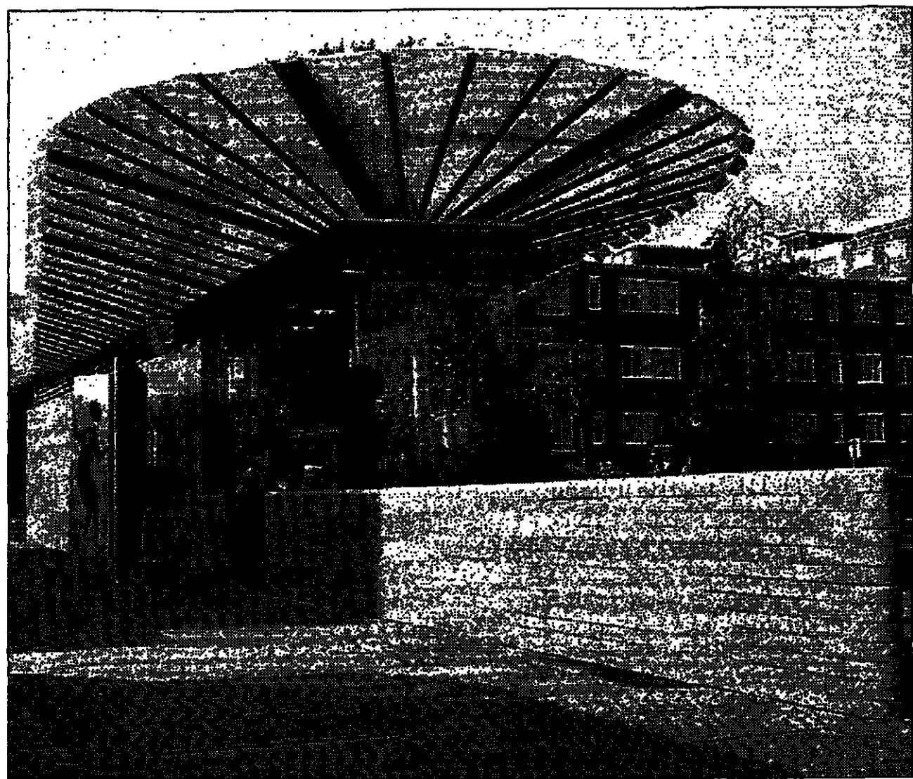
Piers Gough's landmark loo in the London neighborhood of Notting Hill, complete with a florist's kiosk.
